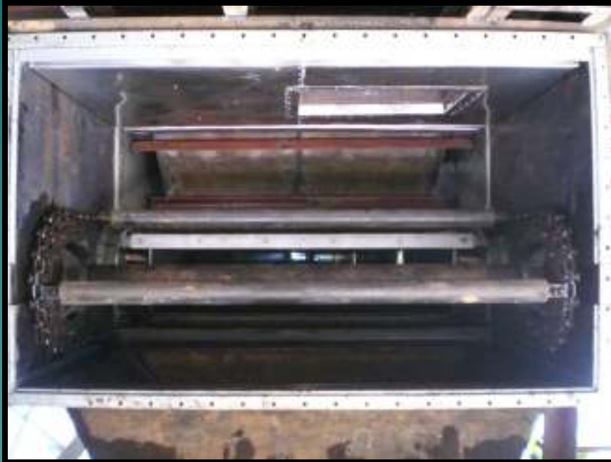
EXISTING DRIVE SHAFT
