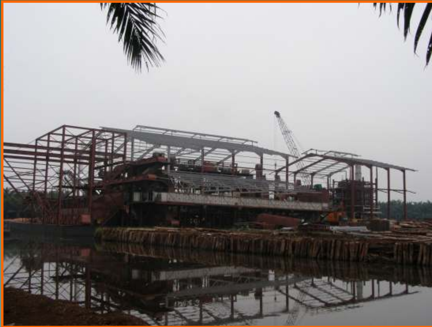
PALM OIL MILL – 30 TPH (UNDER CONSTRUCTION)
