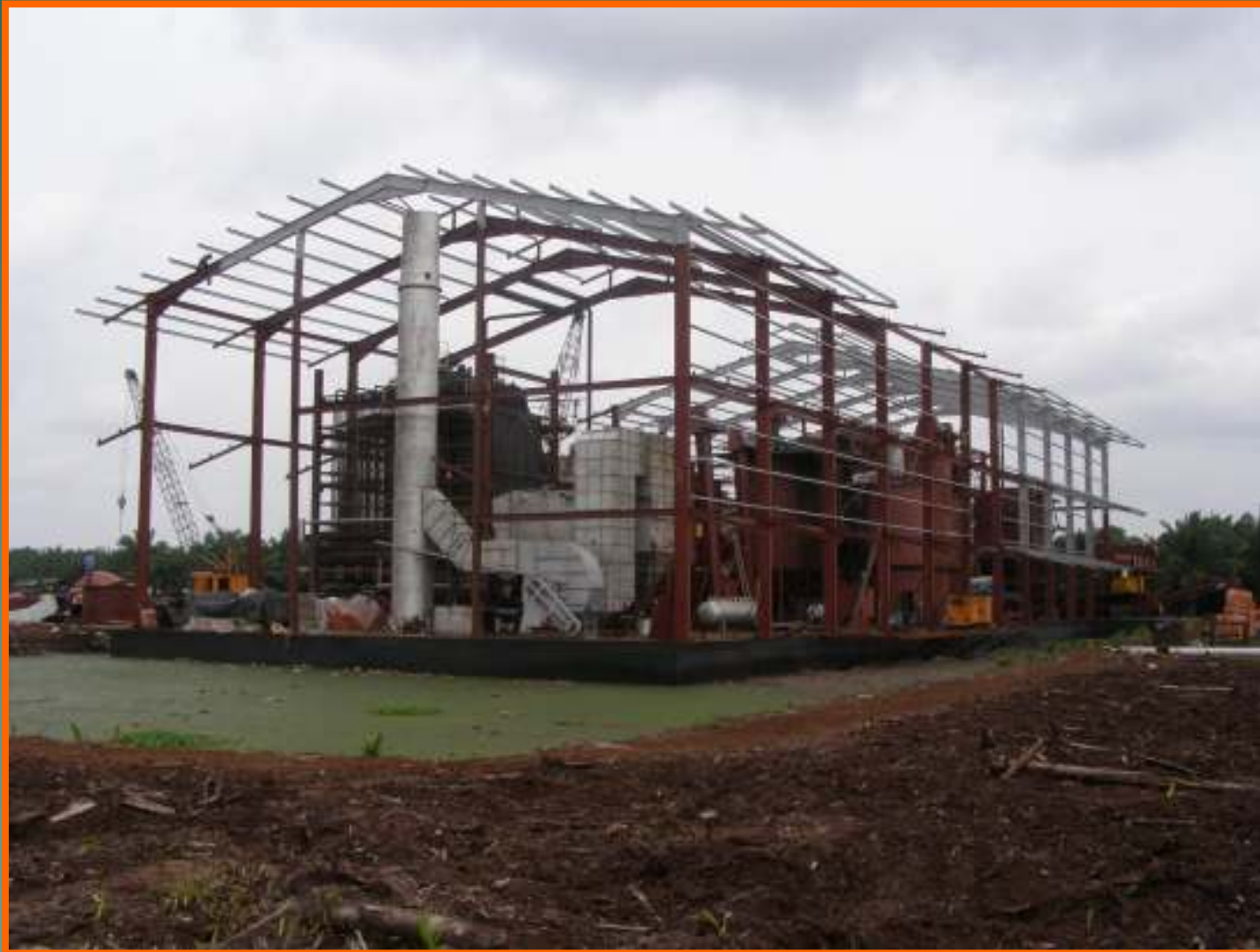
PALM OIL MILL – 30 TPH (UNDER CONSTRUCTION)
